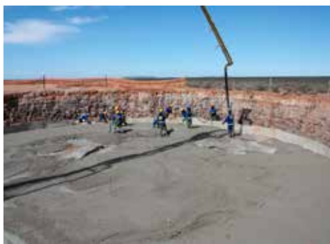
Each one of the 61 bases uses 353 m 3 of concrete.
