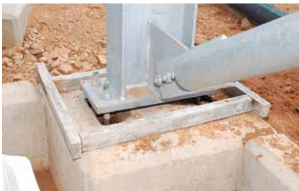
Grouting preparation.
