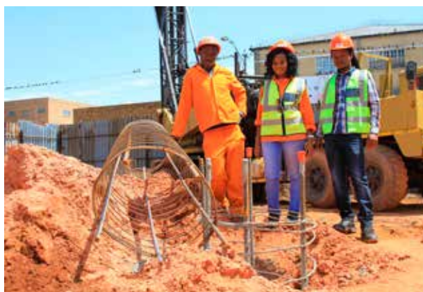
Ernest Makwala, site foreman; Keo Lekutu, contracts manager; and Sibongiseni Dlomo, health & safety officer, with a reinforcing cage for one of the 54 foundation piles.
