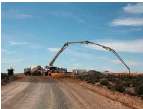
Pouring of concrete under way.
