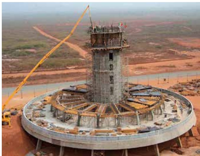
Constructing the control tower at Dakar International Airport, Senegal, using ULMA formwork.
