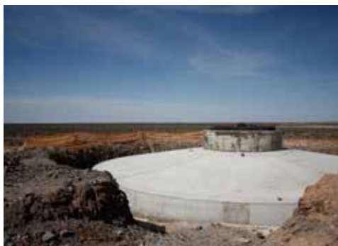
The 61 plinths of the Loeriesfontein Wind Farm were constructed using 1,500 m 3 of high-strength 60-MPa concrete comprising 75% GGCS.
