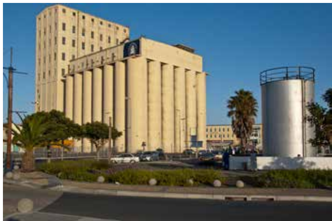
The historic Grain Silos before work began. Credit: www.traveller24.news24.com
