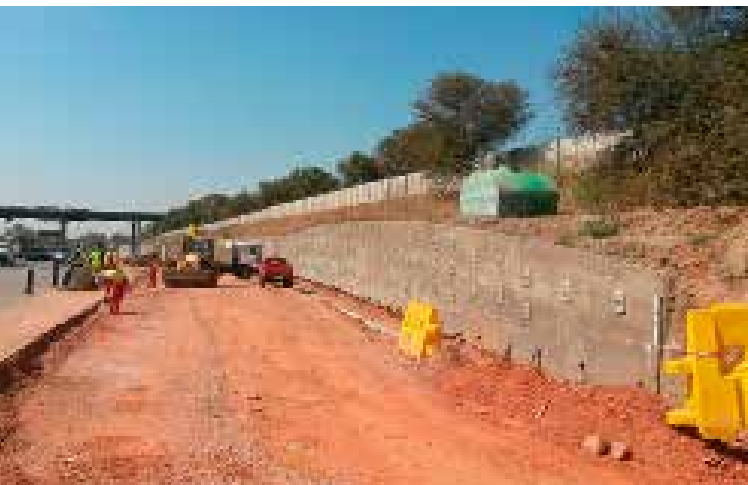
Construction of a concrete retaining wall using shotcrete.
