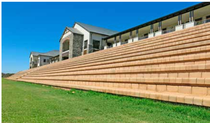
The Reddam House installation of Terraforce's 4x4 seating system.
