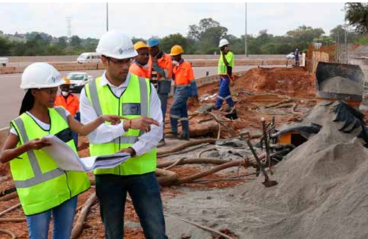
Construction underway on the Zambesi Plaza upgrade.
