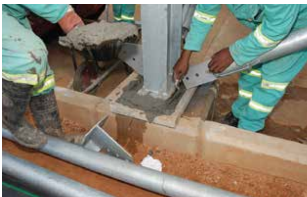
Grouting in progress.
