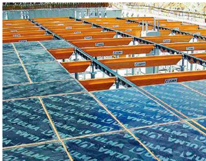
Aluminium decking system CC4.
