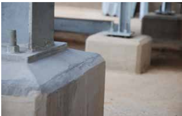
Grouting completed and dry.
