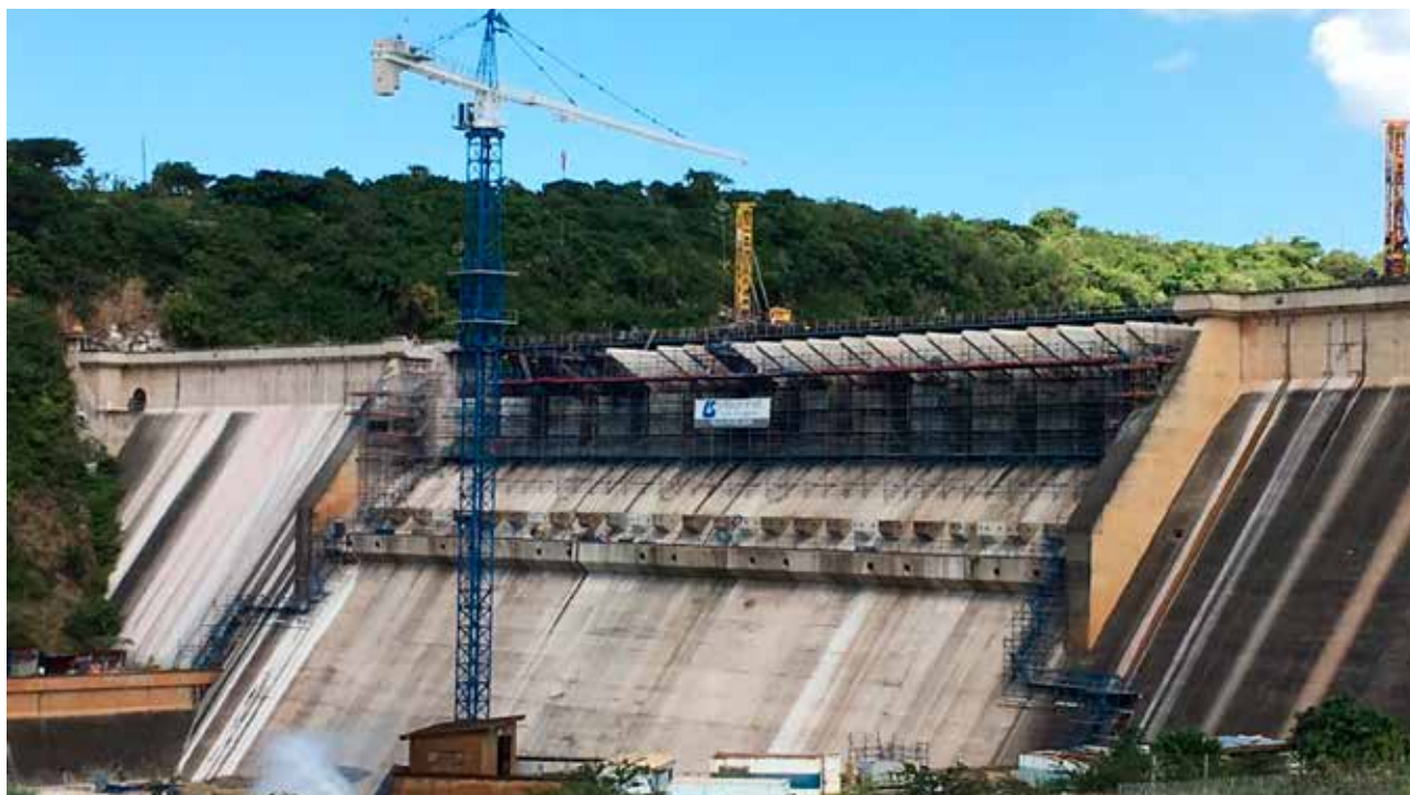
Overall construction of the Hazelmere Dam expansion to raise the dam wall by seven metres. A total of 83 anchors will be inserted along the entire dam wall.
