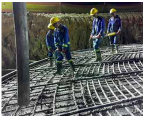
Two bases were poured using high-strength 45-MPa concrete comprising 80% waste to ensure the necessary strengths could be achieved.
