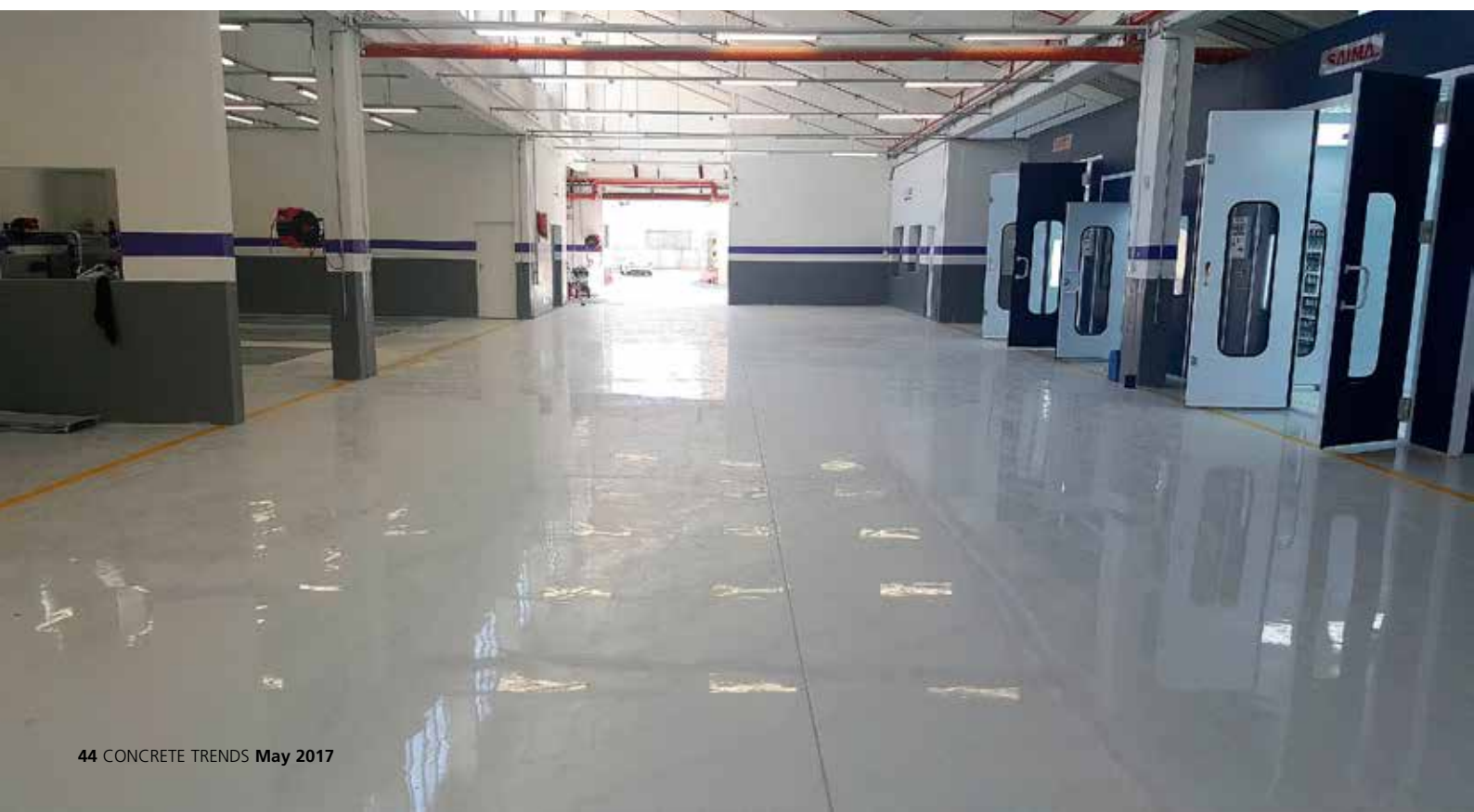
a.b.e. Construction Chemicals' abecote 400 Hi-build flooring system was applied to new floors at Tekton Autobody Repairs in Paarl.
