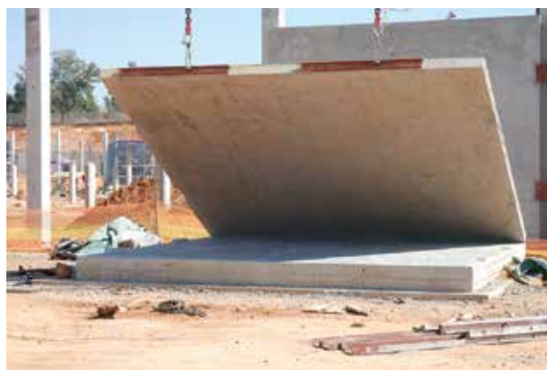
Stack casting panel being lifted off stack.
