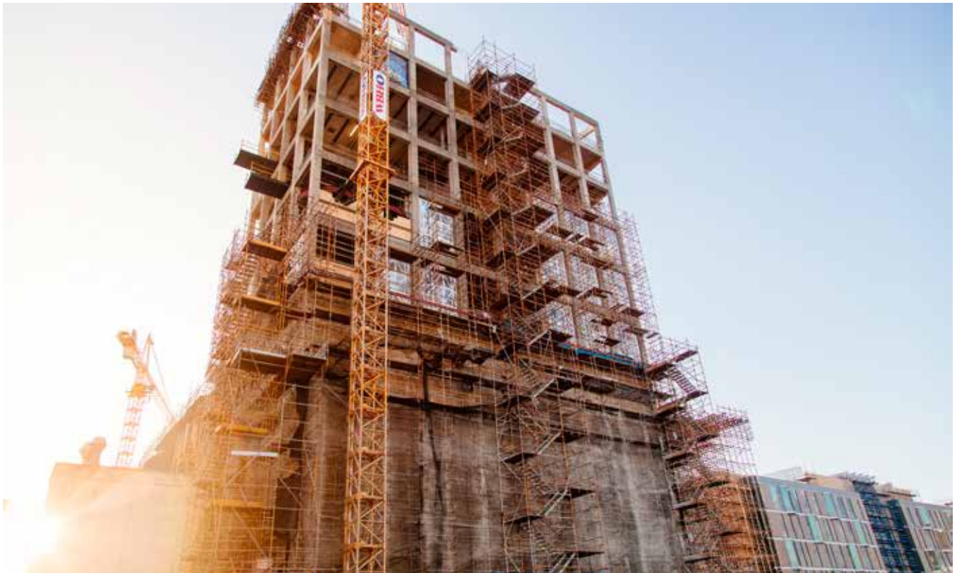
The elevator building forms part of atrium, and a transfer beam had to be formed on the sixth level of the east side of this structure. Credit: Grant Duncan-Smith.
