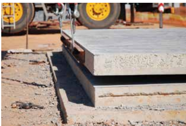
Stack cast separation using release oil.
