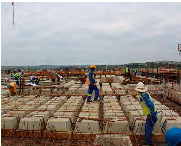
AfriSam readymix has been used for the slabs, suspended slabs and columns.
