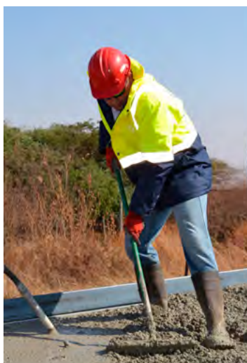
Placing concrete on site.
