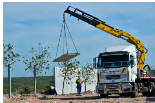
A Topfloor wall slab is offloaded prior to installation between the steel H sections.
