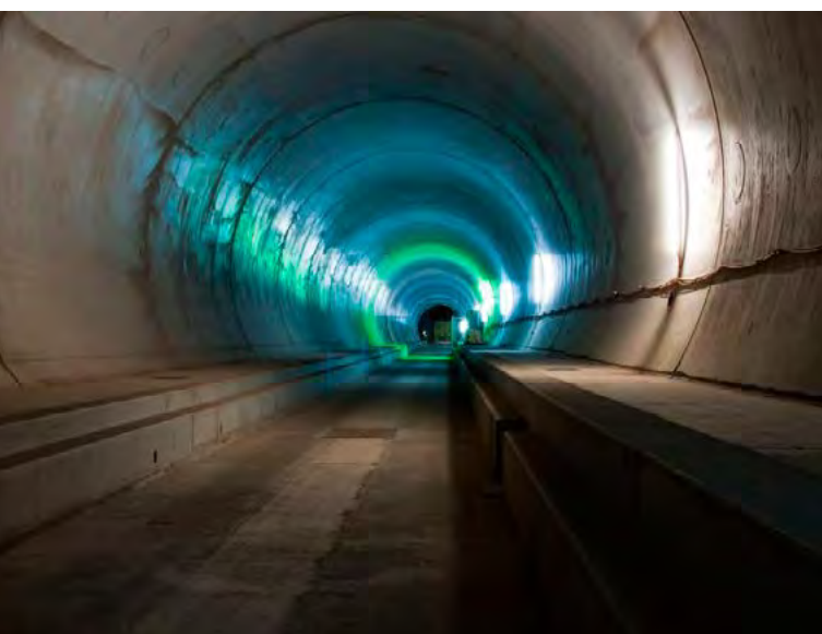
Straight and flat, the GBT clears a major traffic bottleneck through the Alps.
