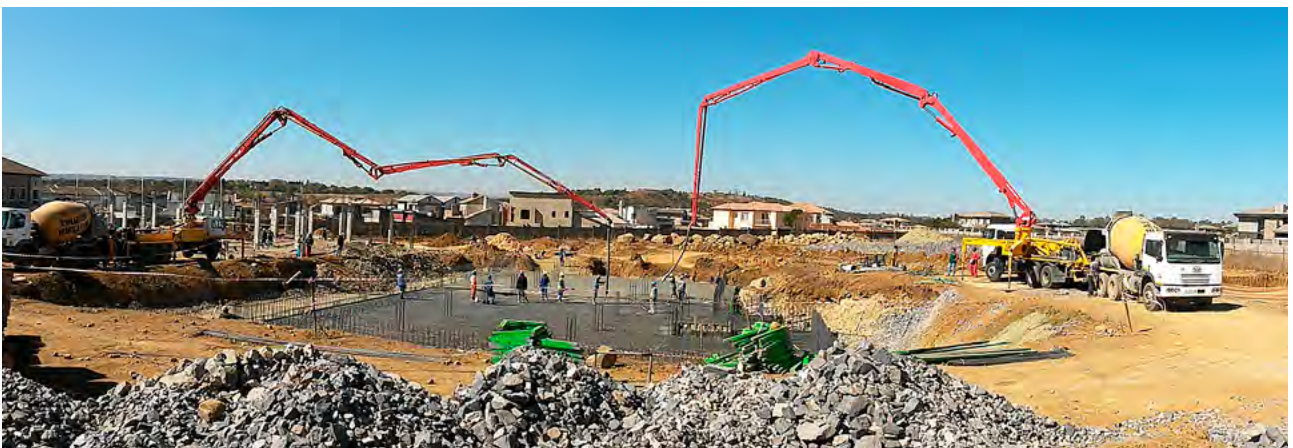
A large raft foundation was used to support one of the two new office blocks built by J.C. van der Linde & Venter Projects at Hazeldean Office Park.
