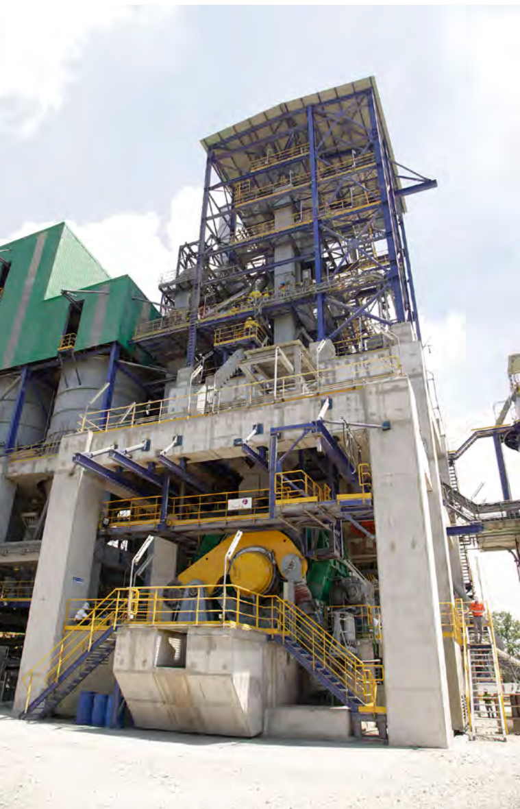
The Teresa grinding plant
