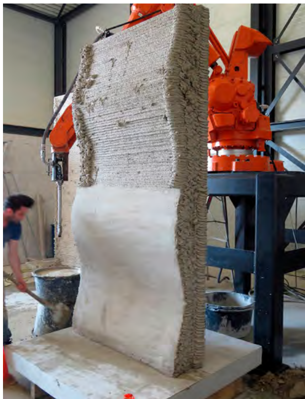
This formwork has a straight and a double-curved side, the bottom of which was given a smooth finish.
