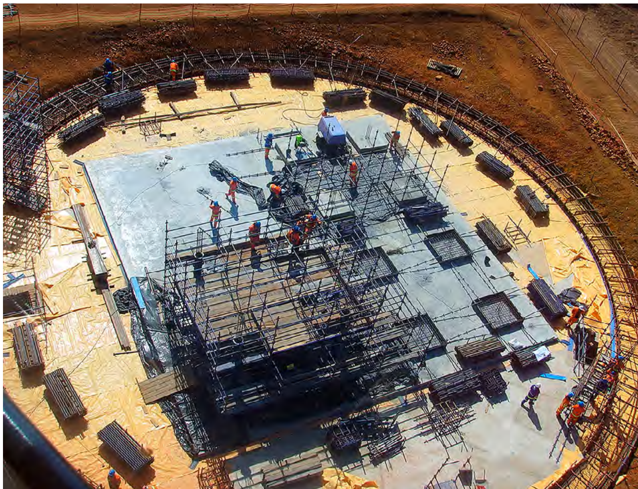
Work in progress on the new concrete reservoir at Savana City in Sebokeng.
