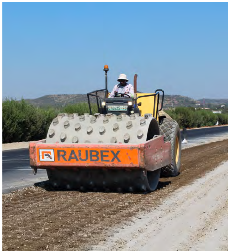
Raubex is stabilising the sub-base to a depth of 350 mm with AfriSam's Roadstab 32.5N CEM II B-L cement.
