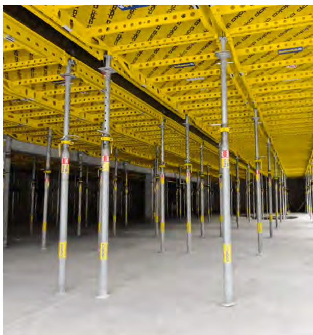
Wide spacing of props creates plenty of working space.
