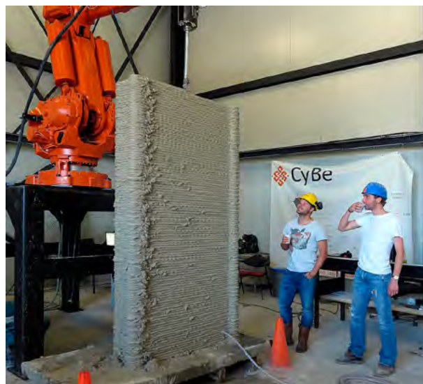
The first 3D print was a hollow formwork (1.25 metres wide, 35 cm deep and 3.1 metres high), which was filled with water to establish the maximum 'formwork load'.
