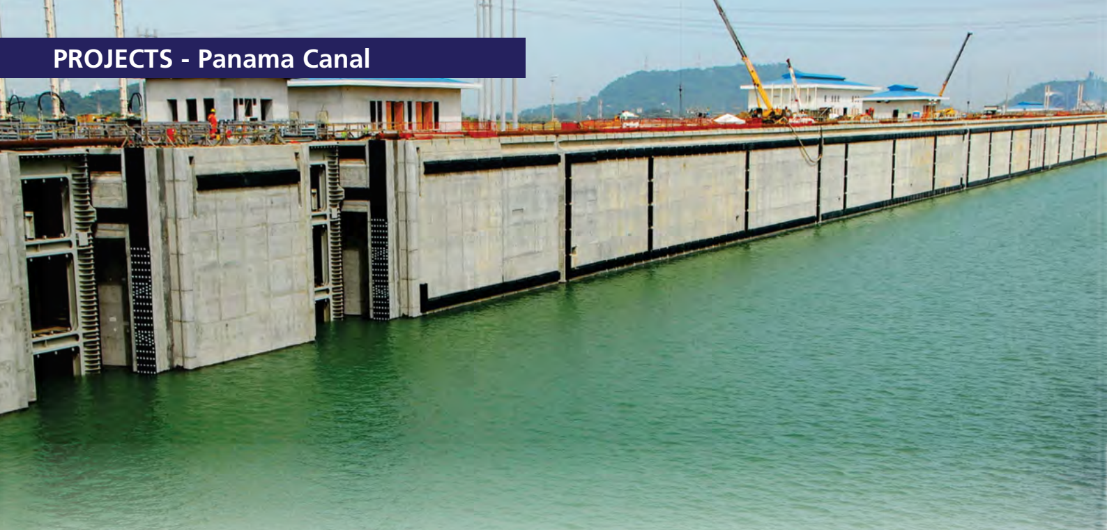
One of the locks in the completed Panama Canal Extensions.
