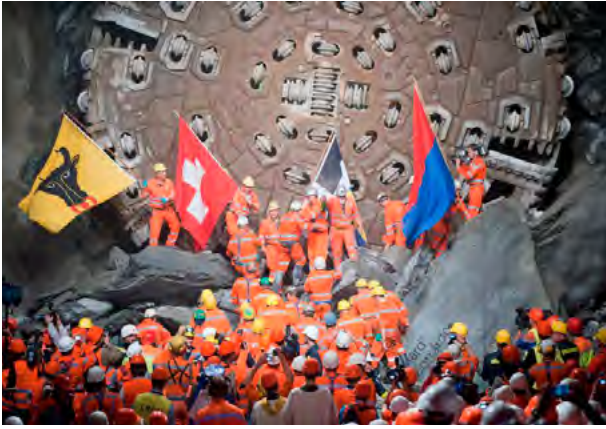
The tunnel breakthrough occurred in October 2010.
