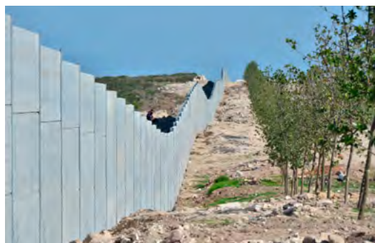
A section of completed security wall built with Topfloor prestressed hollow-core slabs at the Saldanha Naval Base.
